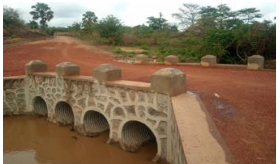
Abele to Nyangilia road opened and 4 lines of culvert bridge installed
